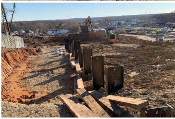
Pictured From Top to Bottom: Rendering of the Residences at North Hill Development; Building pad 2A stabilization with geopiers; Retaining wall soldier piles in place with lagging ready to be installed.
